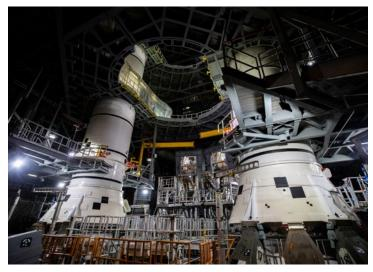
The solid rocket boosters' aft assembly includes the aft skirts with thrust vector control system inside that helps steer SLS during ascent. The entire weight of the SLS rocket goes through the aft skirt structures.
