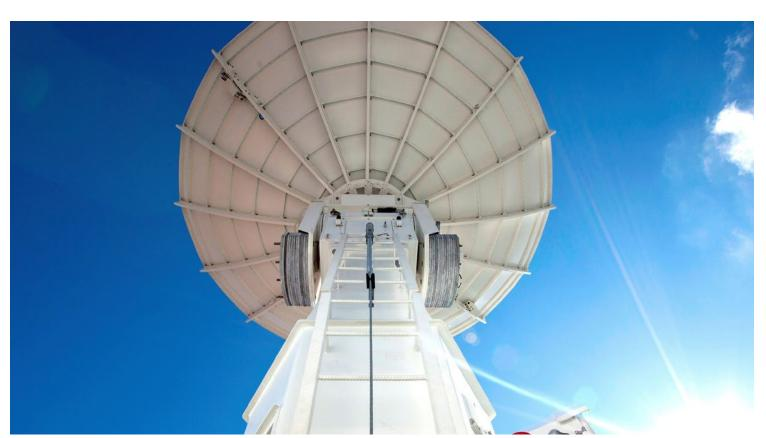
Part of the Kennedy Uplink Station, the S-band ground tracking system at Kennedy provides crucial tracking and communication capabilities following liftoff of SLS and Orion.
