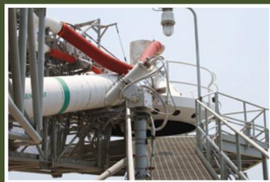
*The Beanie Cap served an important purpose – preventing extremely cold oxygen that vented from the External Tank from turning into ice and potentially damaging the launch vehicle.*
